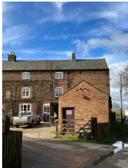
Figure 15: Kingarth Farmhouse is a 3-storey, Grade II Listed structure featuring red brick and Swithland slate.
