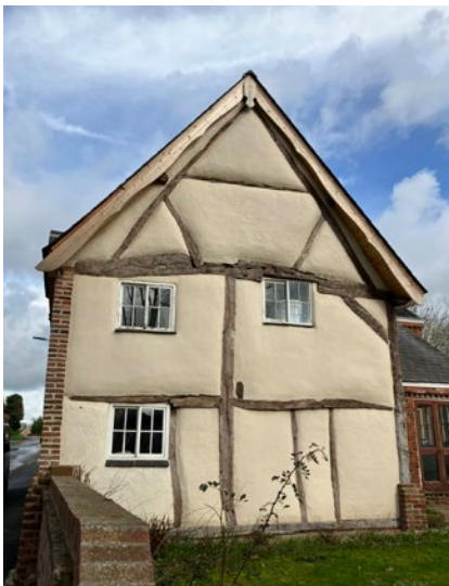
Figure 14: The Grade II Listed Overton Cottage dates from the 17th Century and features a distinctive timber frame.
