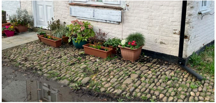
Figure 36: Inset pebbles (here laid in lines running perpendicular to the highway) help to designate the boundaries of dwellings with minimal setbacks along Main Street.
