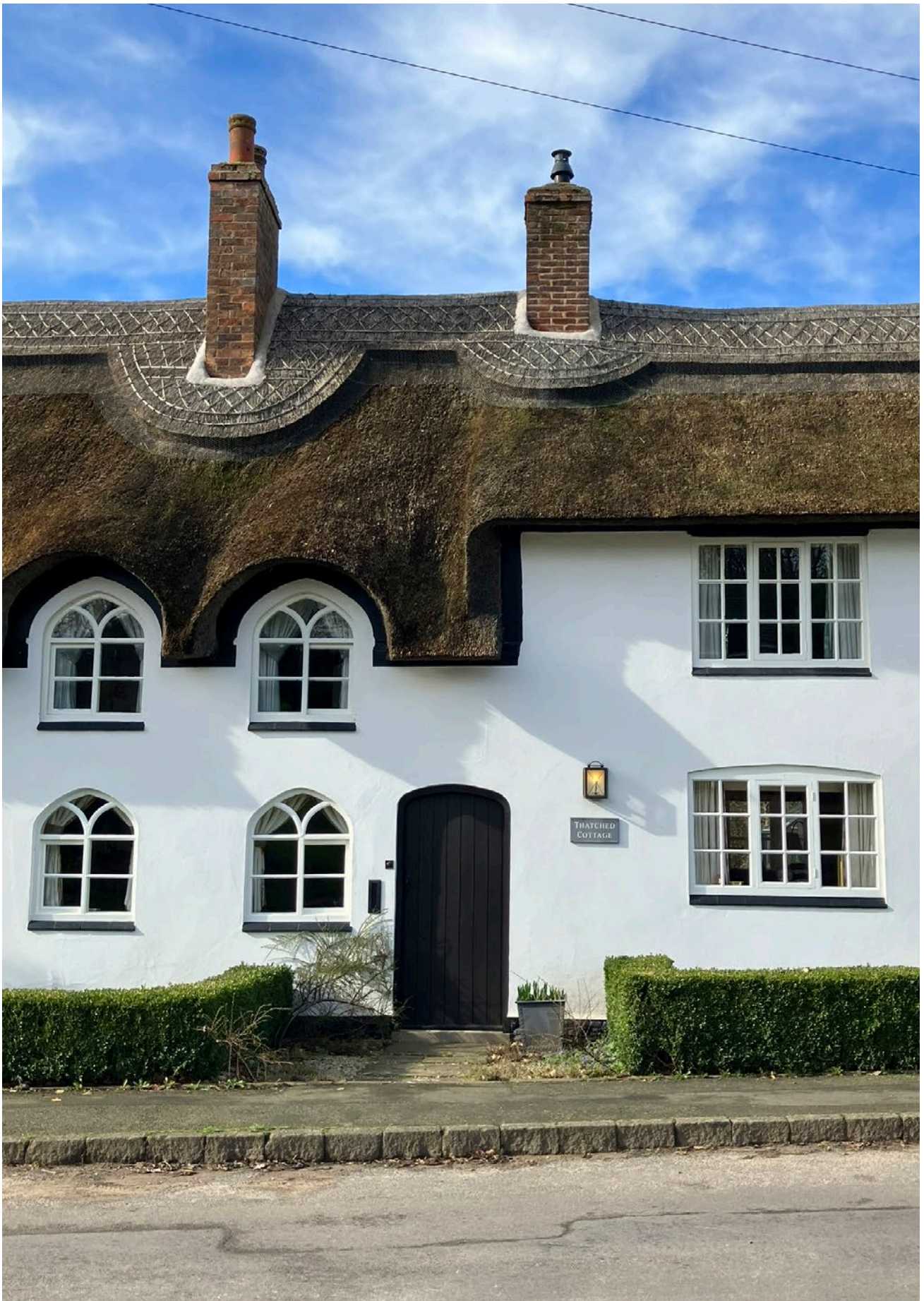
Figure 07: Thatched Cottage, a Grade II Listed building on Main Street, originally dating from the 18th Century. Featuring a whitewashed rendered brick facade and a thatched roof. This 1.5 to 2 storey building has gothic casement windows featuring Y tracery. A small setback from the street with a low hedgerow boundary.
