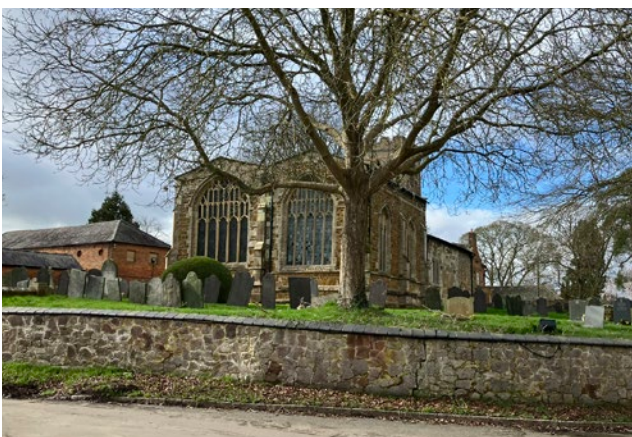
Figure 34: The Grade II* listed St. Andrews Church features ironstone and limestone construction, alongside a granite churchyard wall.
