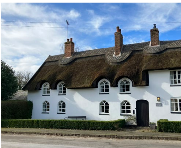
Figure 17: Houses along Main Street are typically 2 storeys, with red brick or white rendered facades. The Grade II Listed Thatched Cottage provides an example of the thatched roofs found in the village.
