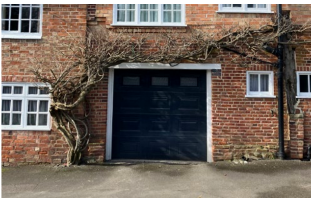
Figure 44: In some historic properties, traditional entrances to courtyards have been converted into integral garages.
