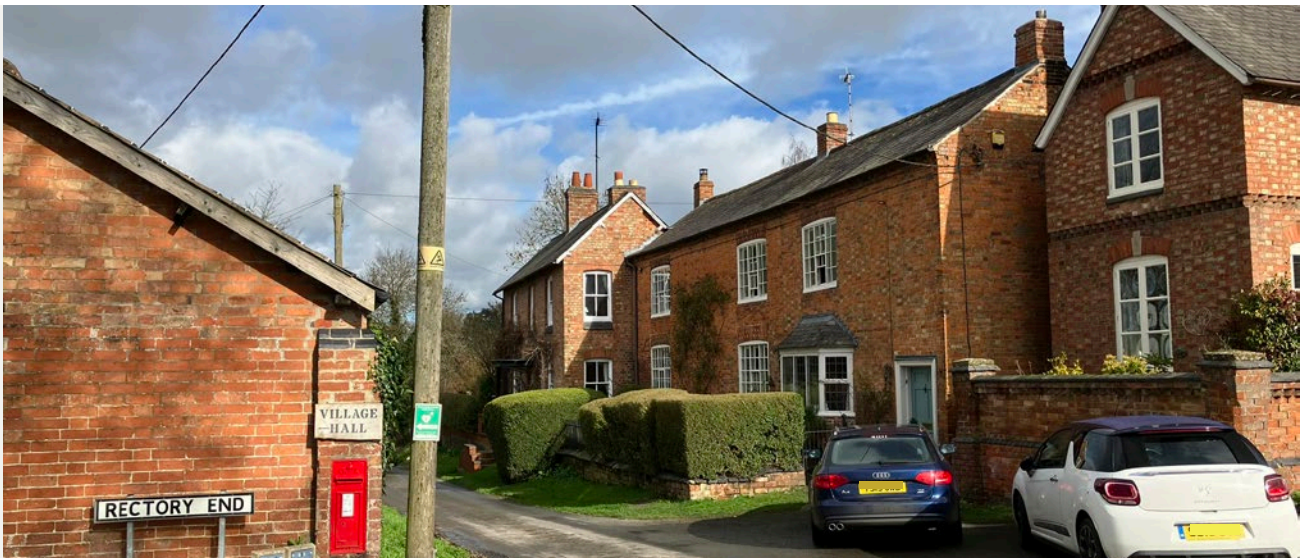
Figure 20: A cluster of red brick buildings mark the corner of Elms Lane and Scotland Lane. All buildings feature curved window lintels, white window frames, and slate roofs - helping them to read as a unified set. Bands of decorative brickwork, alongside alternating hedgerow and brick wall boundaries help to give each home an individual character.
