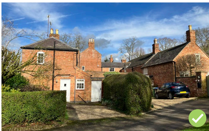
Figure 71: Within this set of converted farm buildings, on-plot parking has been provided within the courtyard created by the U-shaped building layout. This successfully screens the parking from the street.
