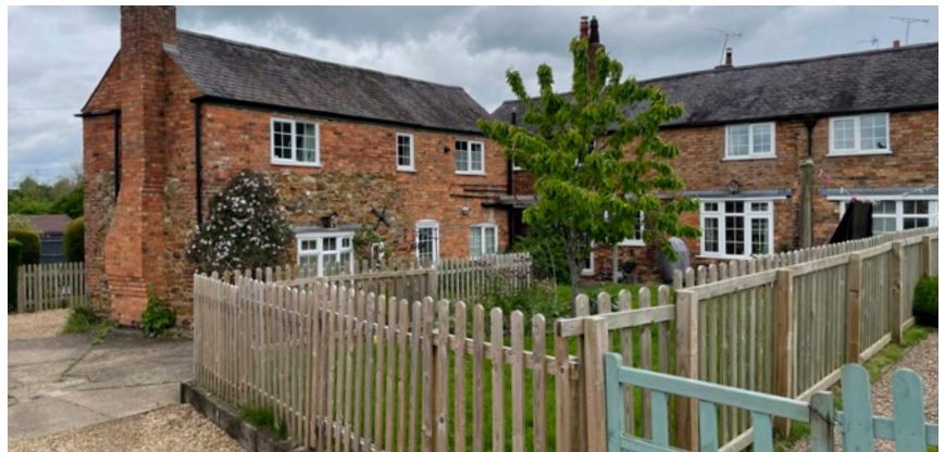
Figure 42: Reflecting its agricultural history, clusters of converted farm buildings with central courtyards are also common in Burton Overy.
