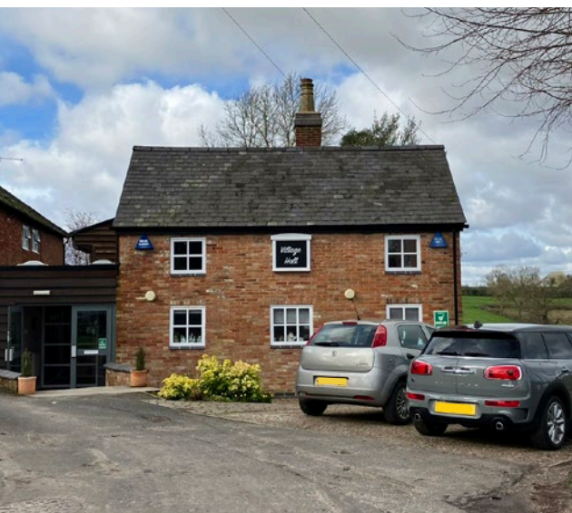
Figure 24: Burton Overy Village Hall is located adjacent to St. Andrews Church and is a key community asset. Comprises two former C18 cottages.
