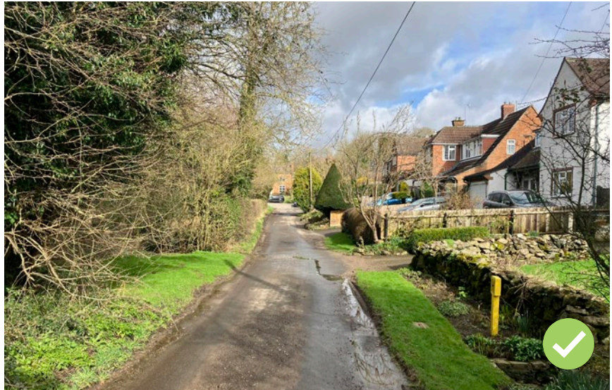
Figure 80: A good example of edge development in Burton Overy where building frontages face outwards onto the surrounding landscape. Hedgerows and mature trees also screen the development, retaining the visual quality of the landscape.
